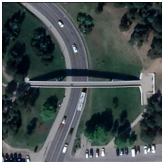
Figure 35. Bridge where measurements were taken
