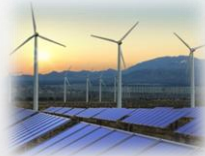
Wind Power Inverters
